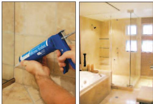
Mildew-resistant silicone for sealing glass-to-glass, glass-to-metal, metal-to-fiberglass joints in frameless showers; tubs; sinks; ceramic tile, cultured marble top to back splash; spas.
