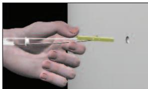
Drill appropriate size hole. Hold metal channel flat alongside plastic straps and slide channel through the hole. Minimum clearance behind wall is only 1-7/8" (48 mm).
