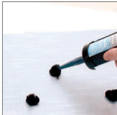
Applying mastic to mirror with Category II Tape applied to back with no holes cut out
