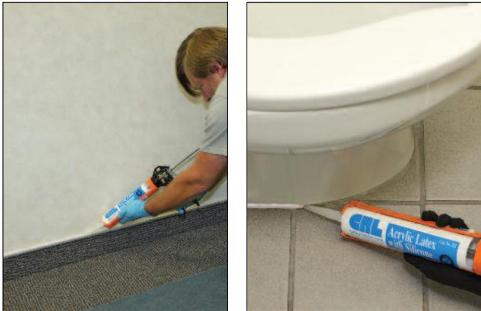
Acrylic Latex Caulk with Silicone for interior gaps around window frames and baseboards; seals around tubs, sinks, back splashes, and toilets.
